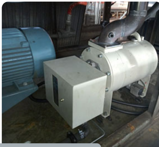
Boiler assembly of the AST preheater K35-50
